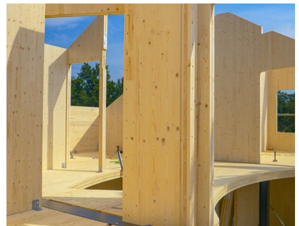
Example of a cross laminated timber building
